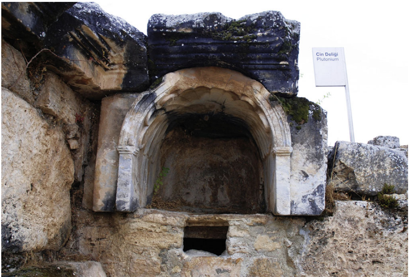
Fig. 5.10 The Plutonium at Hierapolis. Today the entrance to the plutonium is bricked up for safety reasons with only a small opening through which the rushing of the water below can be heard
