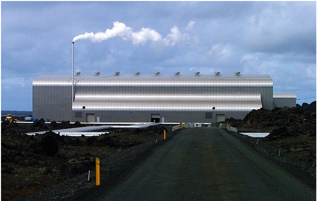
Fig. 11.4 The pioneering Reykjanes Geothermal Power Station in Iceland started to operate in 2006, and since 2009 has the capacity to produce 100MWe 1 using reservoir steam at 290–320 °C. A planned expansion by 30MW is aiming to utilise the geothermal water, which is currently disposed of into the nearby sea
