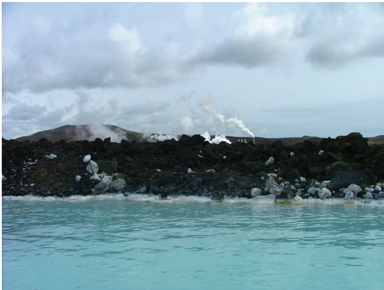
Fig. 1.5 The Blue Lagoon in the south of Iceland with the Svartsengi Geothermal Power plant in the background
