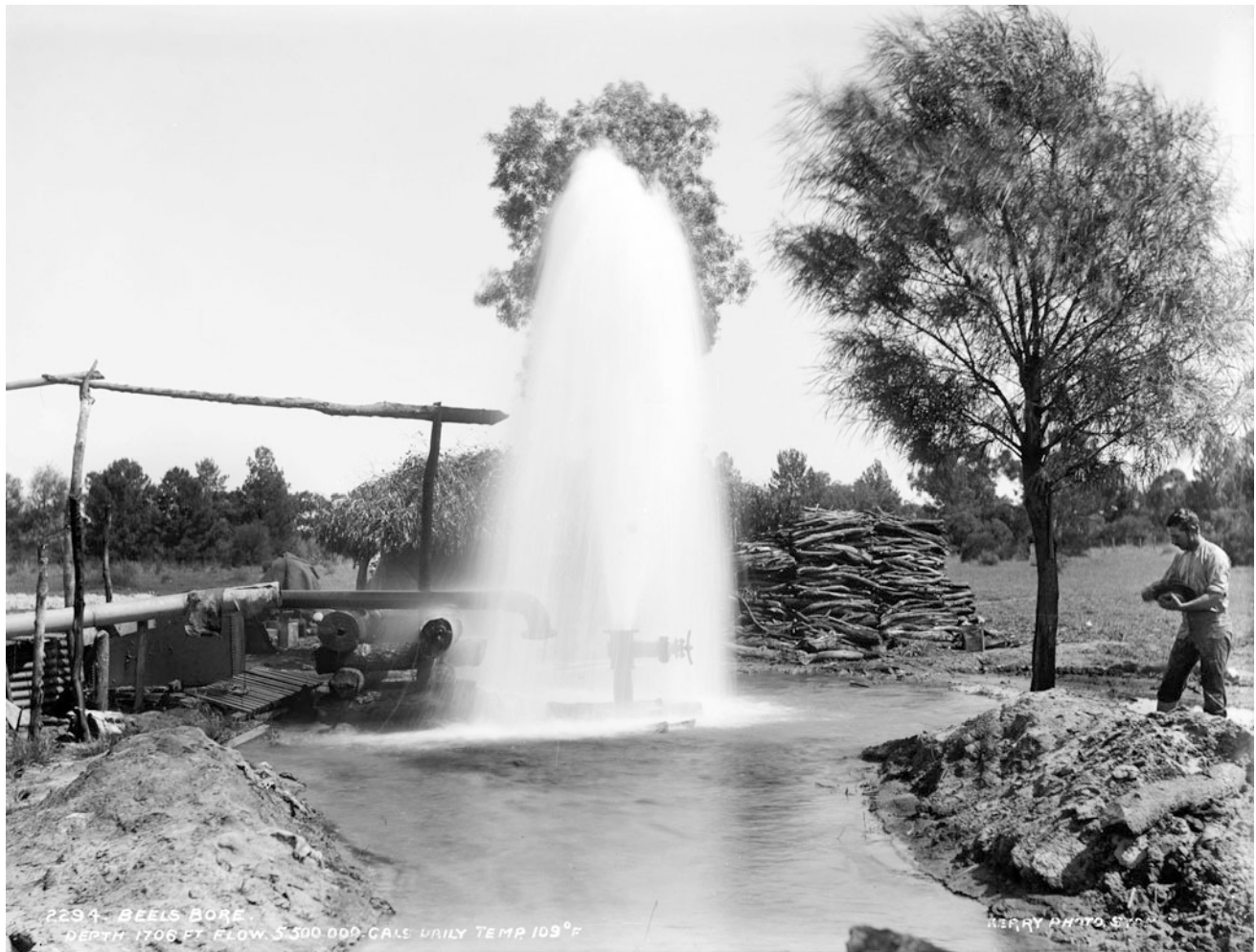
Fig. 2.20 Beel's bore in Cunnamulla, Queensland, was one of the original artesian bores drilled into the Great Artesian Basin underlying much of Australia's outback. At the time, the water from this bore rose
