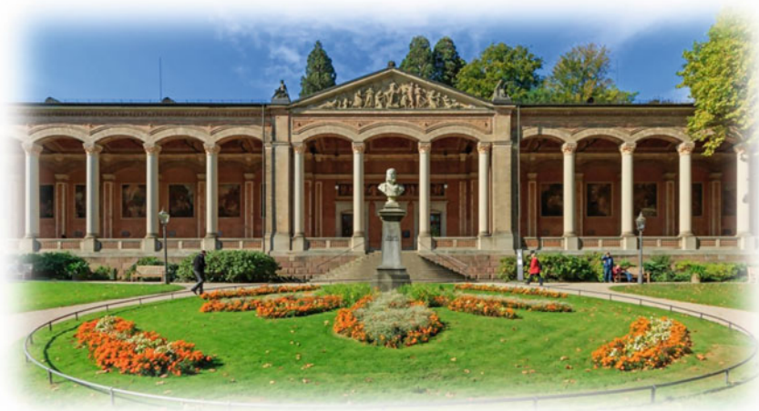
The colonnades and pump house (Trinkhalle) are part of the spa complex in Baden-Baden. Source Alexander Savin (2015b) (Public Domain)
