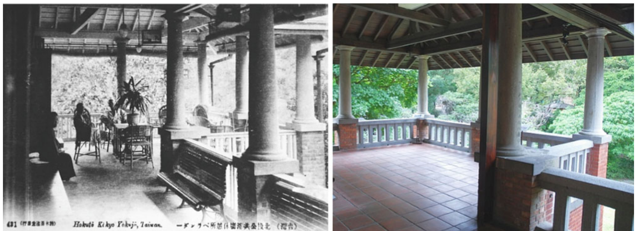
Fig. 9.7 At the turn of the last century the upstairs verandah of the Beitou Bathhouse was an inviting place where people would gather. Now a museum, the same space is devoid of any furniture
