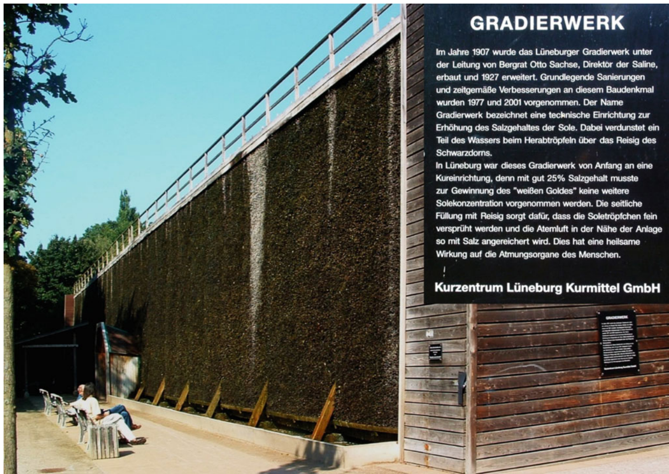
Fig. 8.6 Graduation tower (Gradierwerk) for brine vapour inhalation in the German spa town Lüneburg (Example 8.3; Appendix 8.1). The graduation tower pictured here was constructed in 1907, followed by
